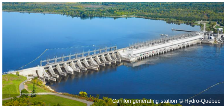
Carillon generating station © Hydro-Québec
